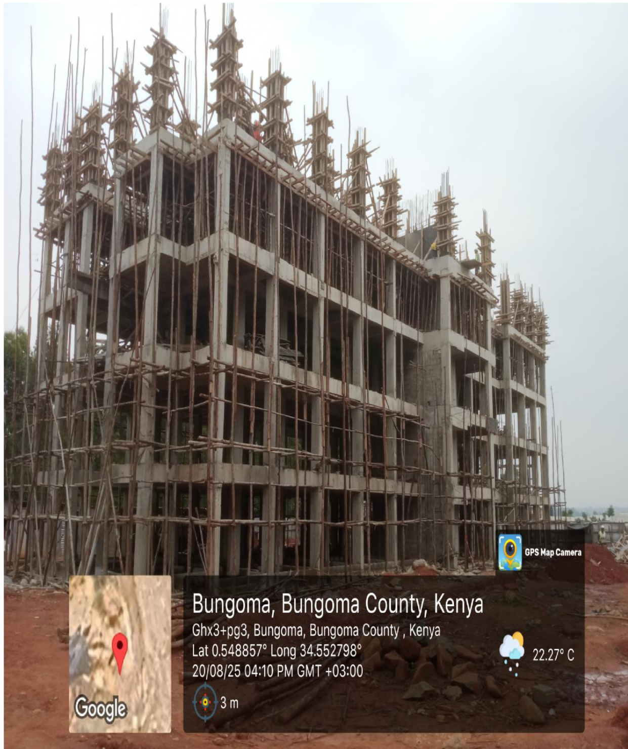
Block C- formwork for 4th floor columns and lift
