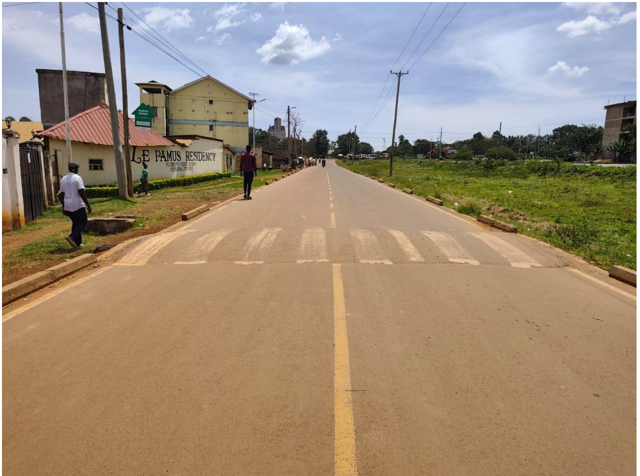
A section of Pamus- Ndengelwa bitumen road in Bungoma town
