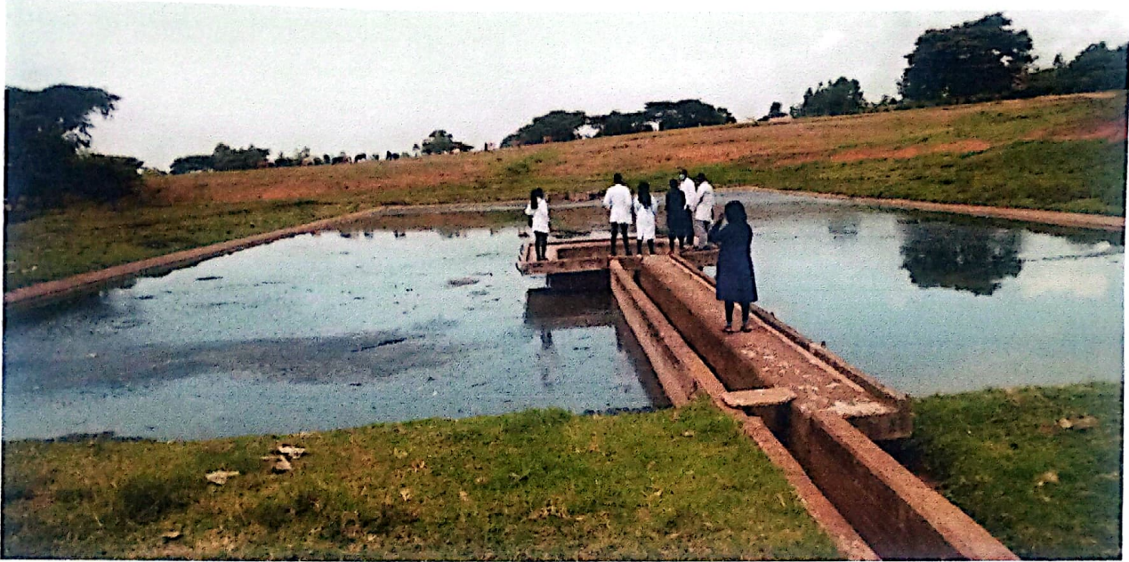
Figure 4 Sewerage Treatment Works(Lagoons) in Khalaba
