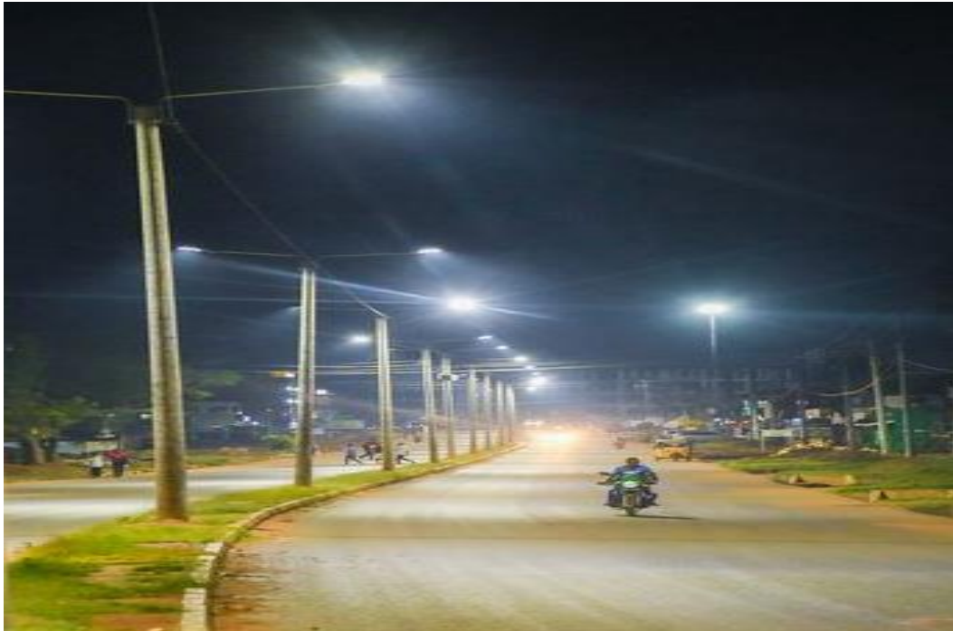
Figure 4: 6.5km Sangálo Junction – Kanduyi Dual carriageway
