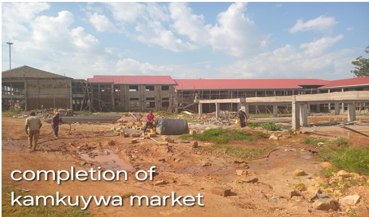
Kamukuywa market under construction
