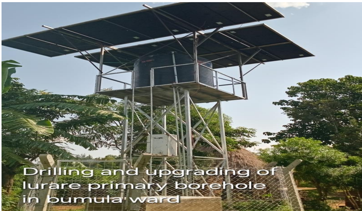
Drilled and upgraded borehole at Lurare primary School in Bumula ward
