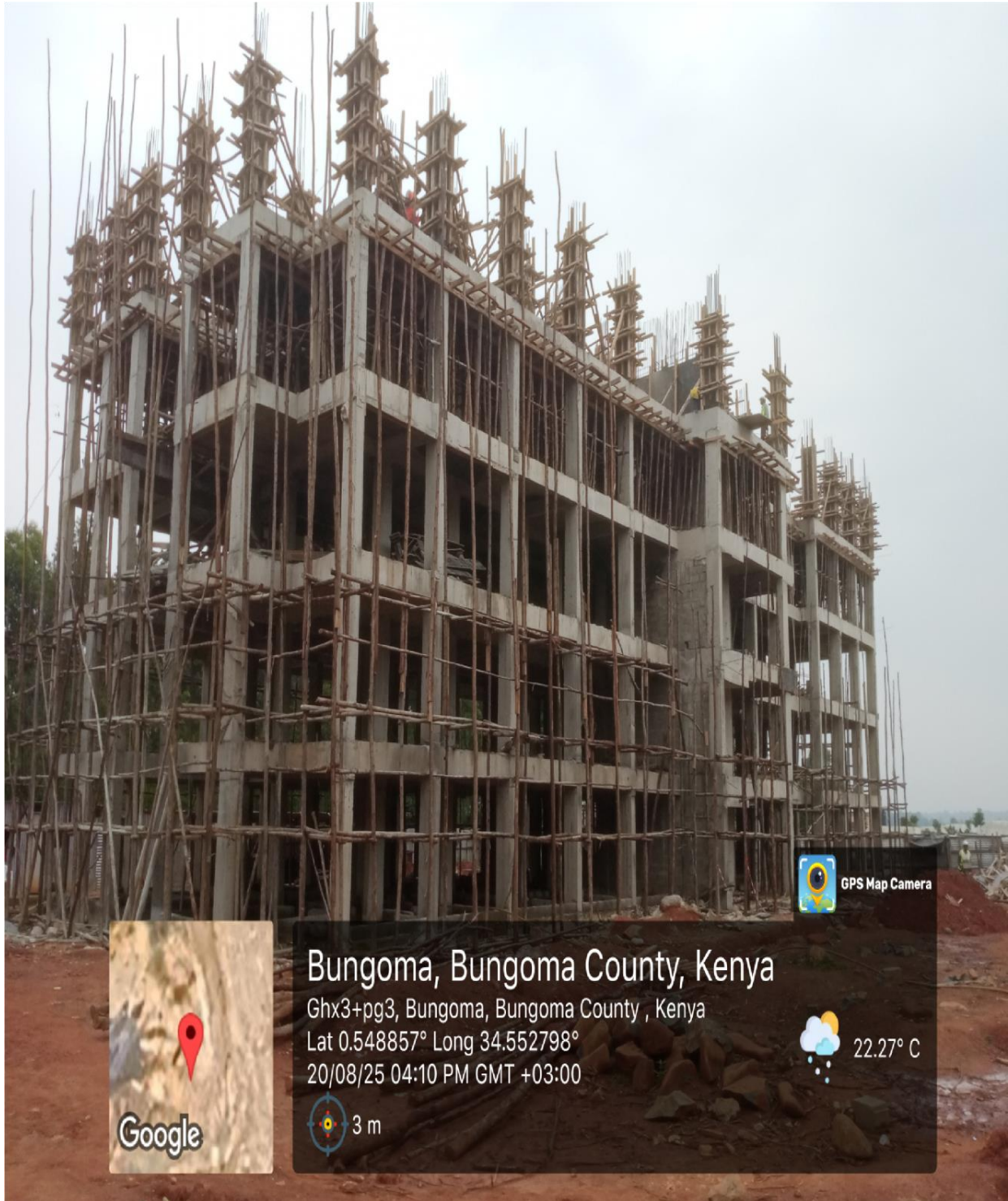
Block C- formwork for 4th floor columns and lift
