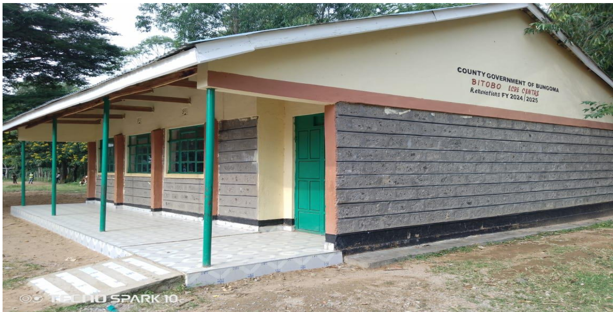
Constructed ECDE classroom at Bitobo Primary School in Kimaeti ward
