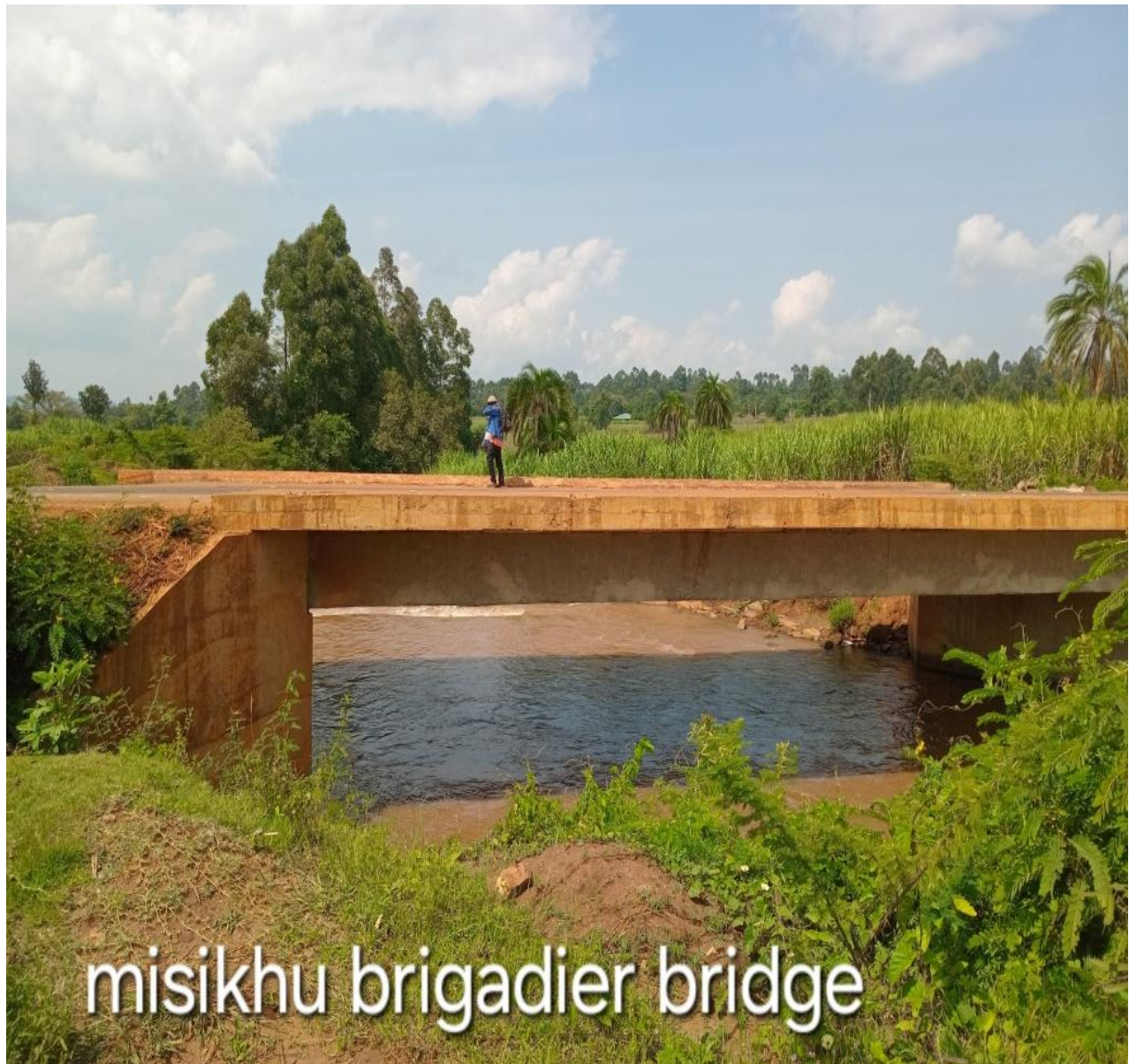
Figure 7: Misikhu Brigadier Bridge
