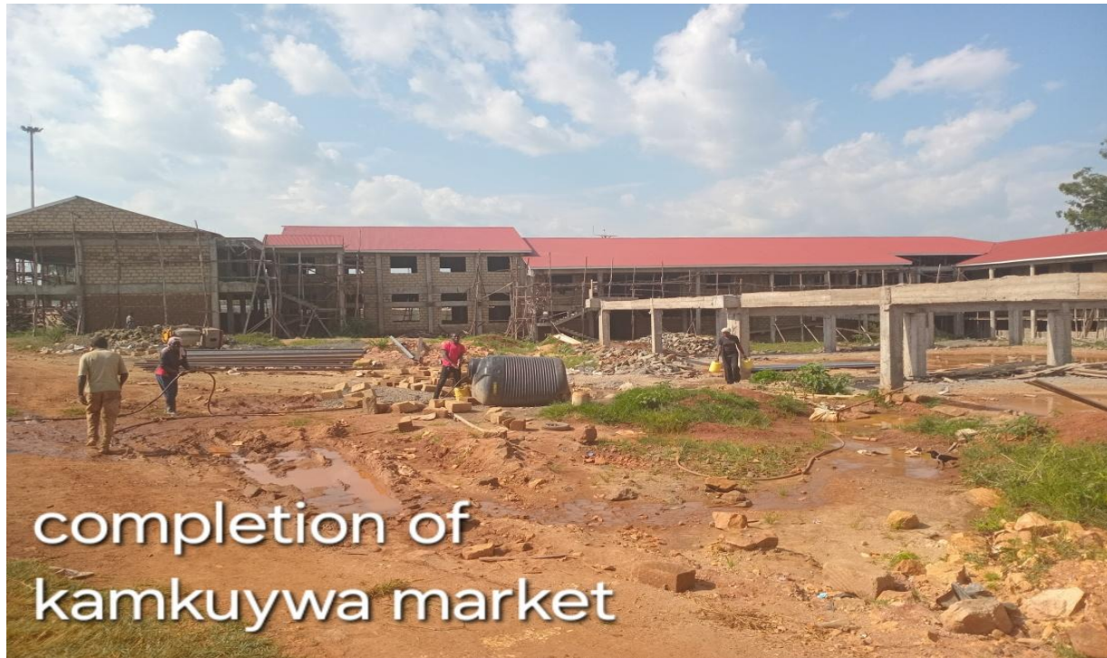
Figure 8:: Kamukuywa Market – Work In Progress
