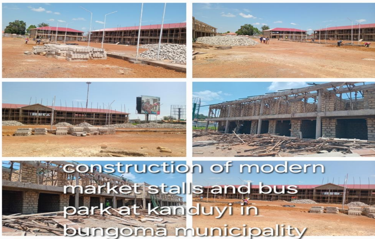
Figure 9: Market Stalls and Bus Park at Kanduyi – Work in Progress
